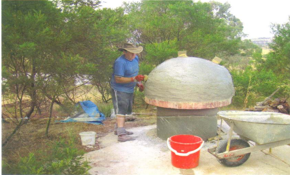
Finishing off with mortar
