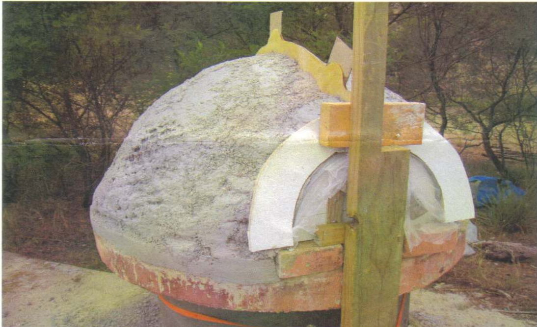
Your advice on mixing consistency was very much appreciated. Netting helped to hold the shape
