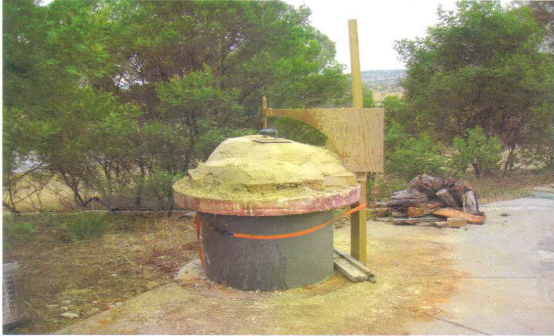
Forming the sand mould. The firebricks are sitting on 20mm of sand. The stand is formed concrete and some scrap 900mm concrete pipe from a local road project.
