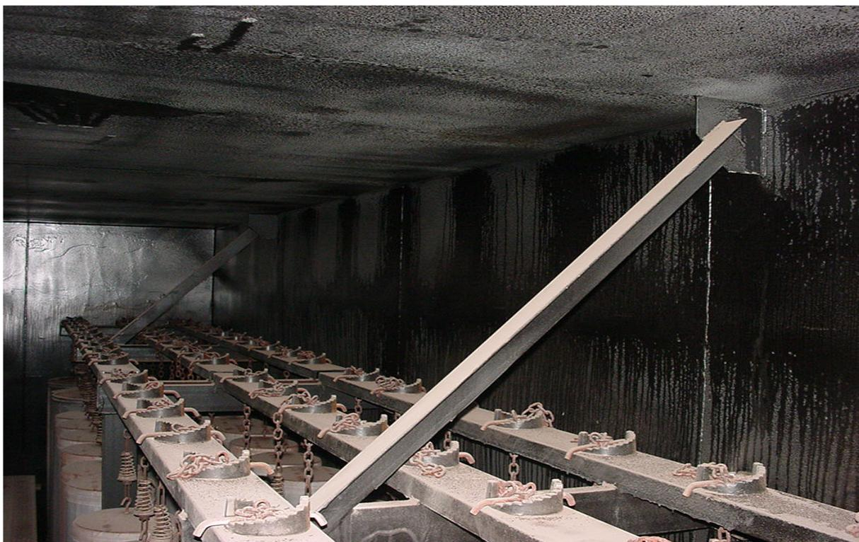
Figure 3. Inspection of coated steel after 2 years in a bag house filter. No corrosion.
