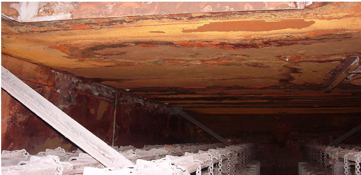
Figure 1. Severe corrosion damage in a reverse air bag house filter
